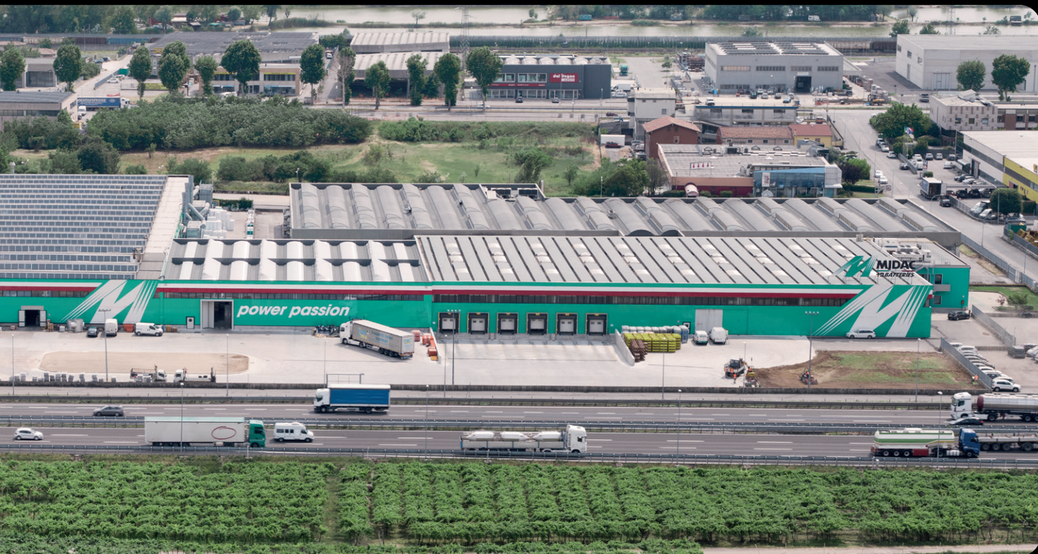
MIDAC HEADQUARTER AND PRODUCTION PLANT - SOAVE, ITALY
