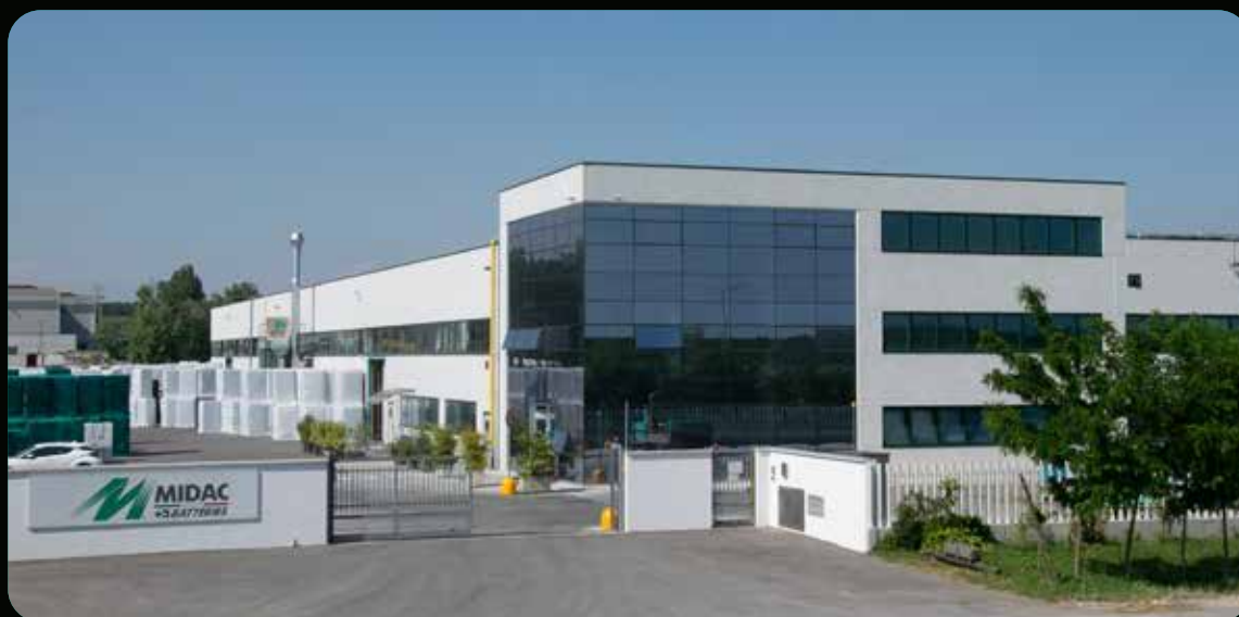
MIDAC 2 nd PRODUCTION PLANT - CREMONA, ITALY
